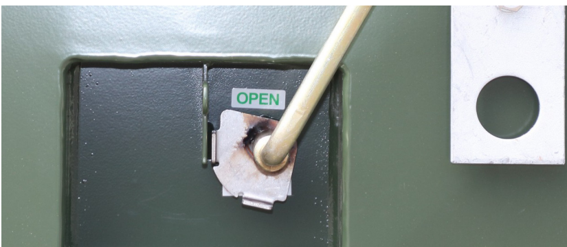
A sturdy operating handle is stored in each operator compartment. The padlocking provisions on the compartment doors accommodate the majority of available padlocks.
